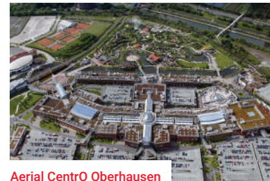
Aerial Centro Oberhausen
